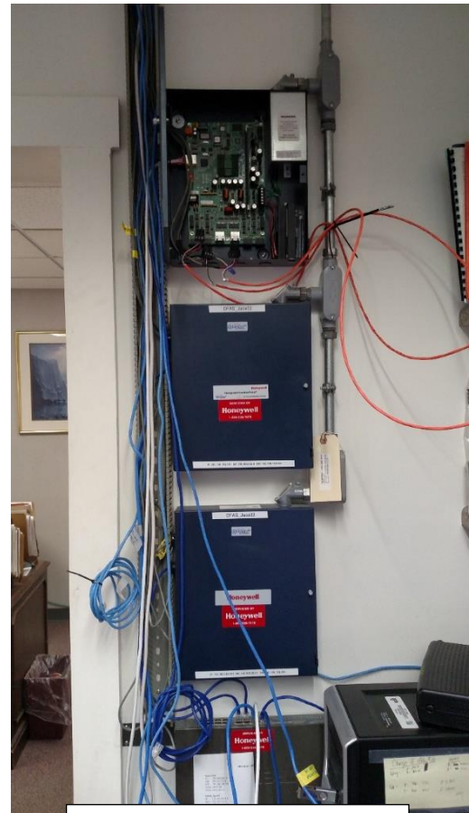
Existing Networking & Wiring
