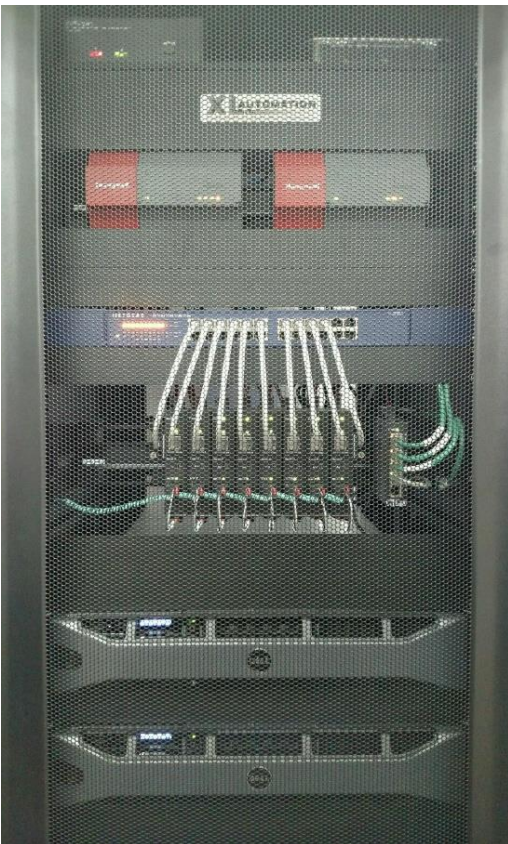
New Niagara Supervisor and network wiring
