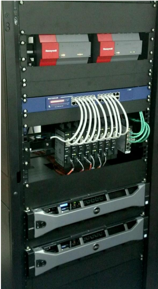
New Niagara Supervisor and network wiring
